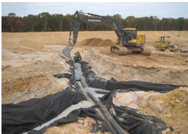
Subcell 9.1 Underdrain Installation
