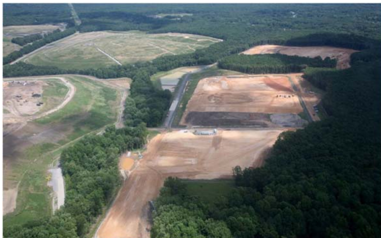
Cell 9 Construction Area
