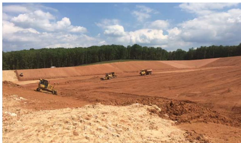
Subcell 9.1 Subbase Installation
